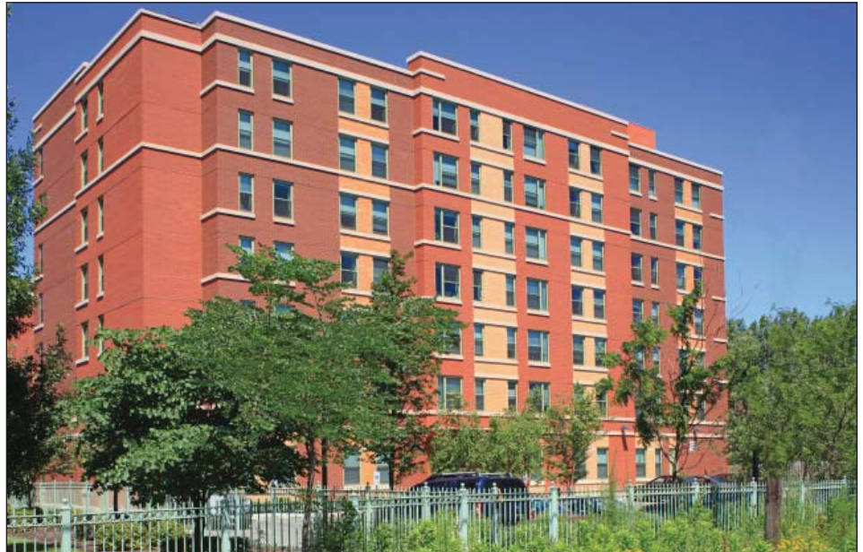
Pilsen's Casa Morelos affordable housing complex completed by McShane Construction Company.
