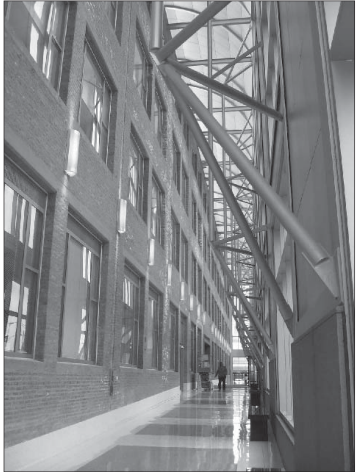
The interior of the Cook County Domestic Violence Courthouse at 555 W. Harrison Street, Chicago, showing the old walls (left) and the new, LEED certified outer walls. The courthouse, completed in 2003, is Cook County's first LEED certified "green" building. It was built by The George Solitt Construction Company, one of many Builders Association companies who have shown a commitment to going "green."
