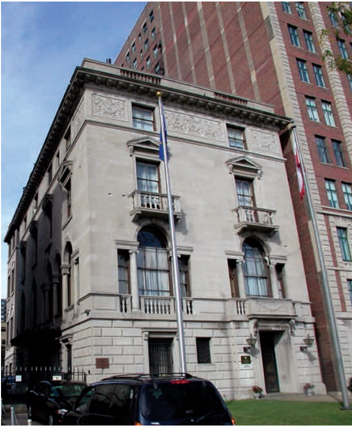
CCOP hires helped the George Sollitt Construction Company build the Polish Consulate.
